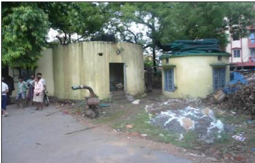
Existing SPS, Saidpur Zone
