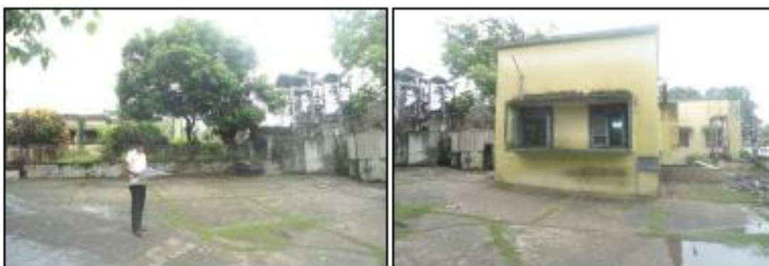
Existing STP, Saidpur.
