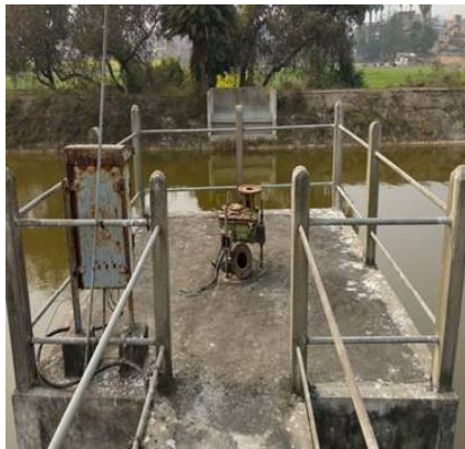
Pump in Aerated Lagoon
