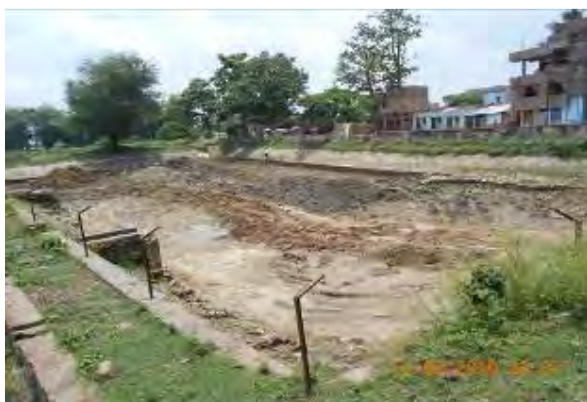
Sedimentation Tank silt removal
