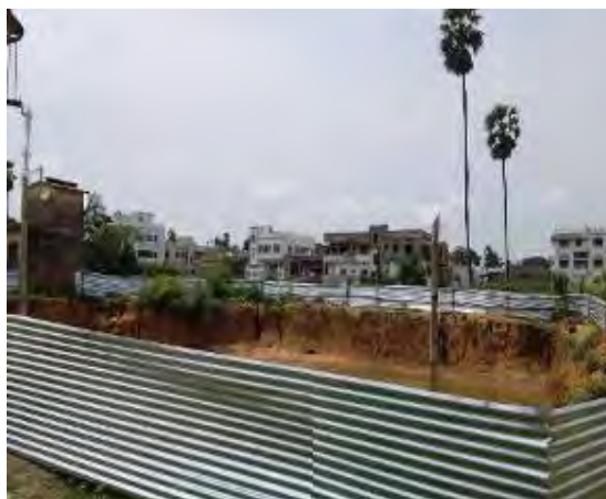
Proper hard barricading
