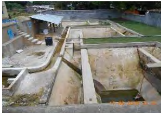
O & M work- Mechanical Filter cleaning
