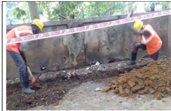
Excavation work is under process for laying pipeline
