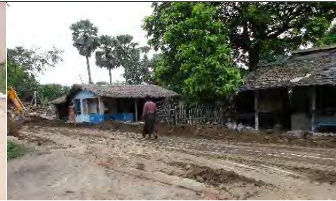
Filling of excavated area after laying of pipeline
