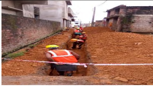
Another view of Excavation work is under process for laying pipeline
