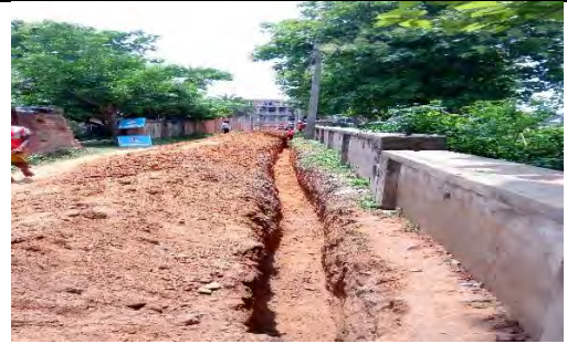
Another view of Excavation work is under process for laying pipeline
