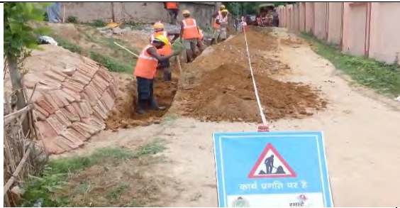
Filling of excavated area after laying of pipeline
