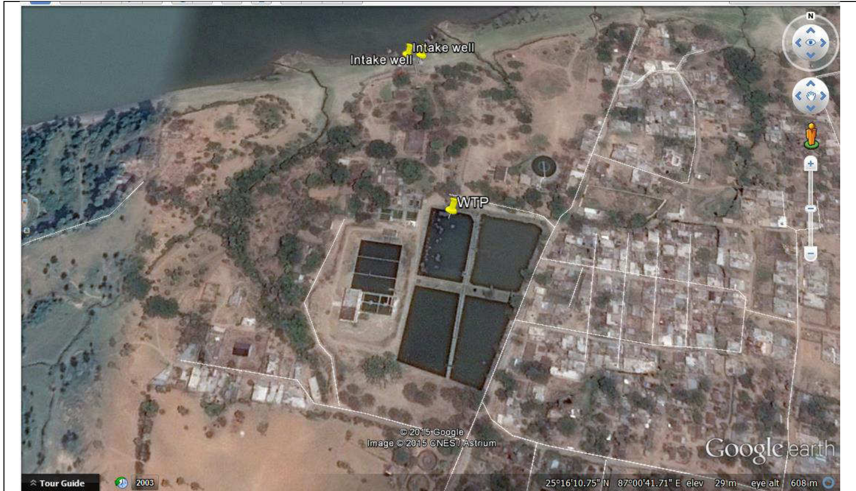
Figure-5: Google Map- WTP Refurbishment at Barari
