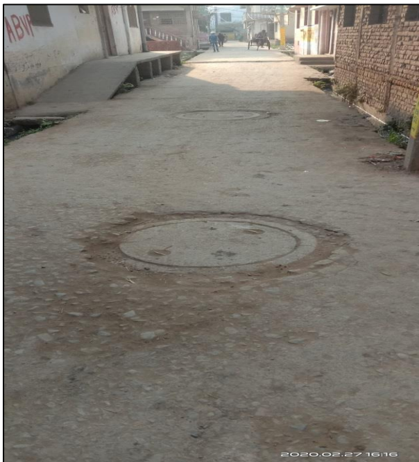
Completed Sewer Network at Ward No. 34 Sugar Mill area Road no.-1
