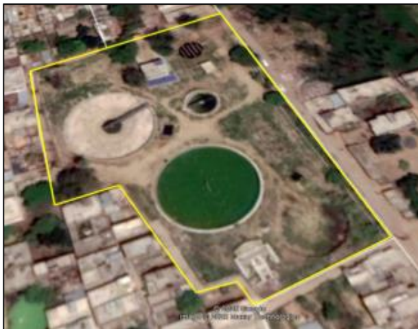
Figure 5-8: Panoramic view of proposed STP site.
